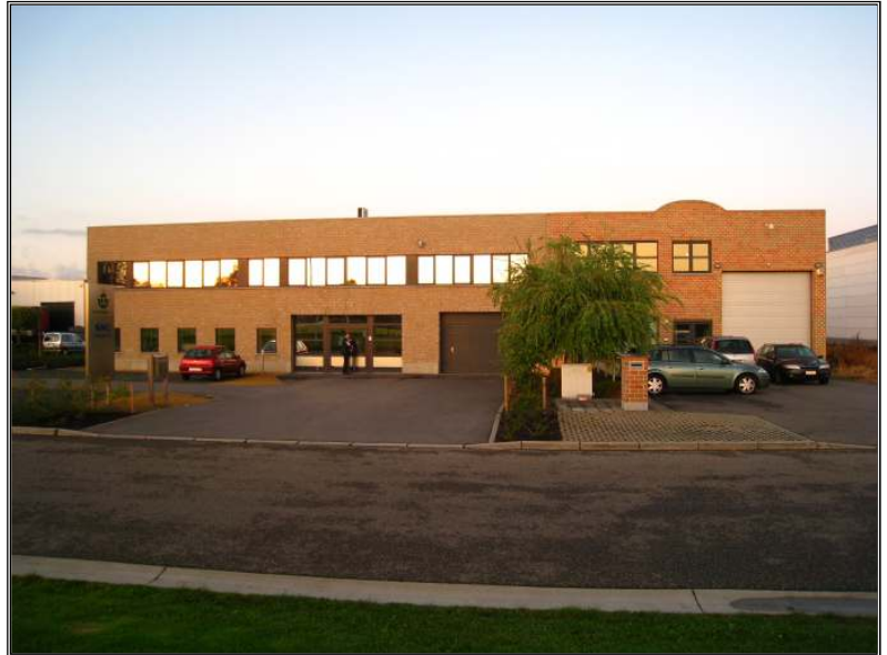
Head Office in Wilrijk/Belgium
